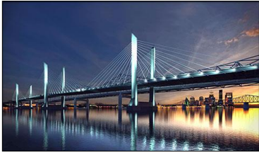
Ohio Precast Concrete Association March 2017 Meeting
